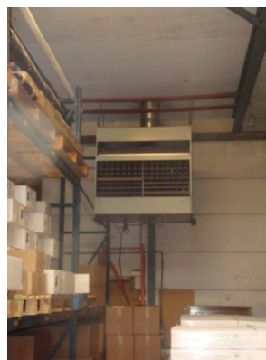
Figuur 3: Direct gestookte heater.
