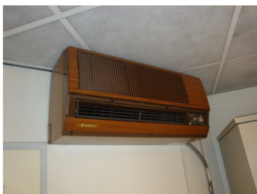
Figuur 4: Wandunit airconditioning.
